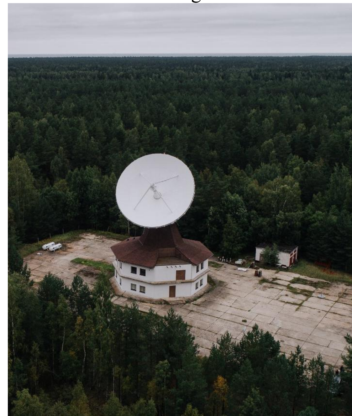
Radio telescope RT-16 16 meters Cassegrain antenna
