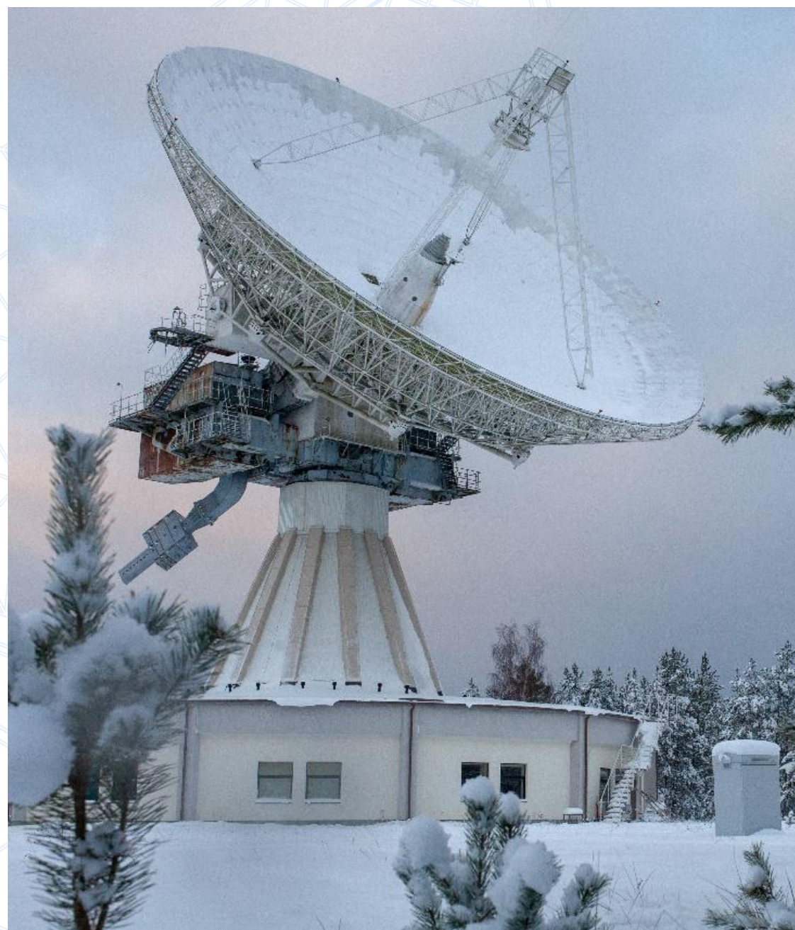
Radio telescope RT-32 32 meters Cassegrain antenna
